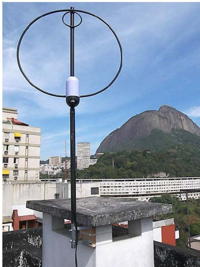
100 watts magnetic loop installed with no holes on the structure.
